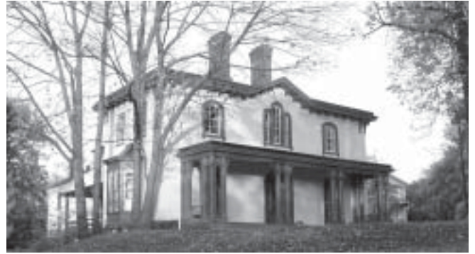
Gray past meets green future... Brentmoor has a state-of-the-art geothermal HVAC system.
