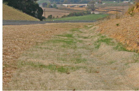
Figure 2: Erosion Control Matting
